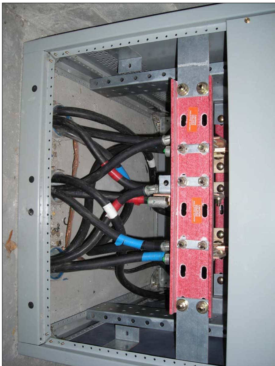
SDS - SECONDARY CONDUCTORS
