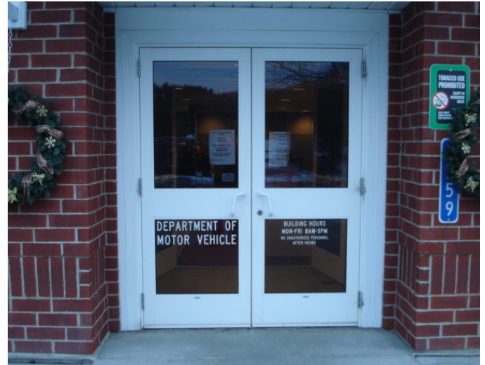
Item 3 doors - Outside view
