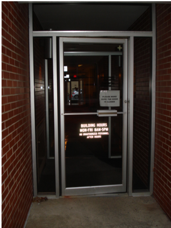
Item 2 doors - Outside view
