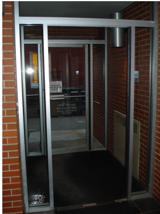
Item 2 doors - Inside view
