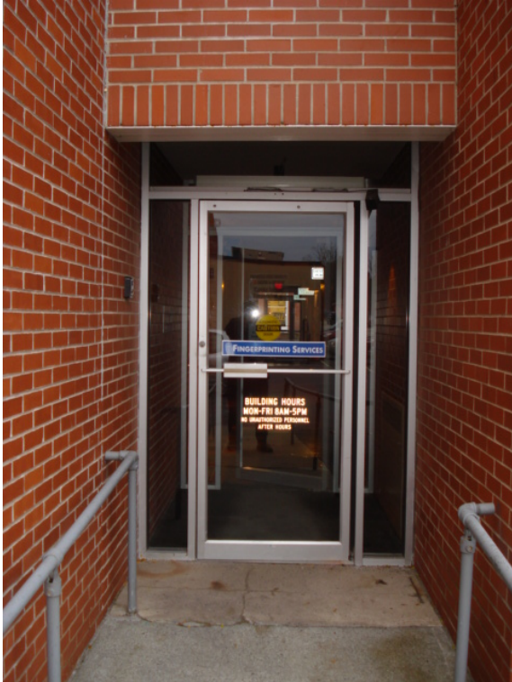
Item 1 doors - Outside view
