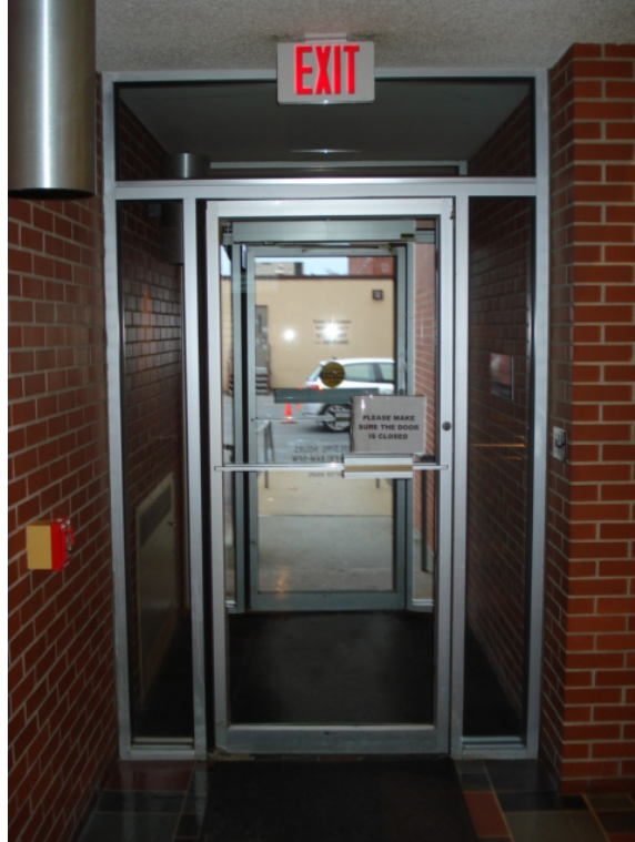
Item 1 doors - Inside view
