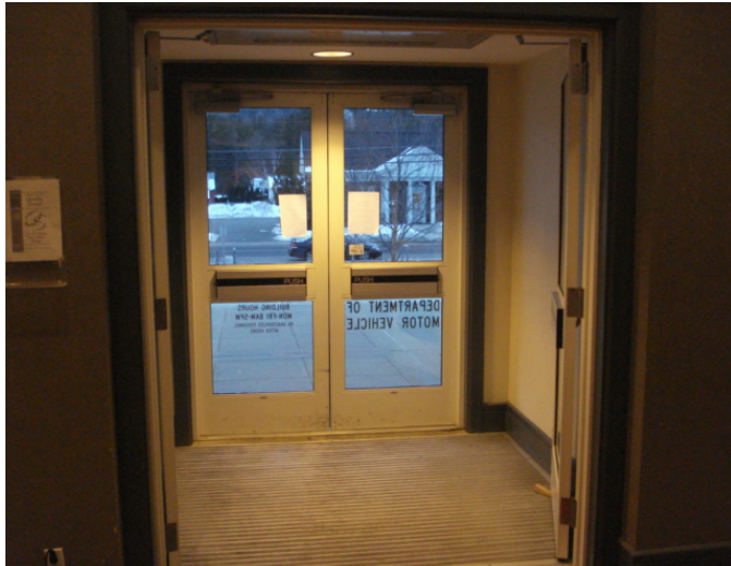
Item 3 doors - Inside view
