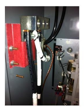
IMG\_1951 is a picture of the generator connections to the Switch. I did put a wrench to the closest ones and they were sufficiently tight.
