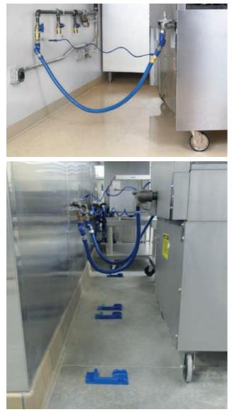
Figure 1 Gas ranges with flexible connectors. Photos courtesy of Dormont Co.
