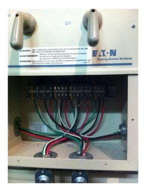
IMG\_1961 is a rough picture of the UPS system layout. UPS load panel to the far right, just out of the picture view. The breaker panel feeds three 20 amp twist lock outlets that power the new Essex County radio racks.
