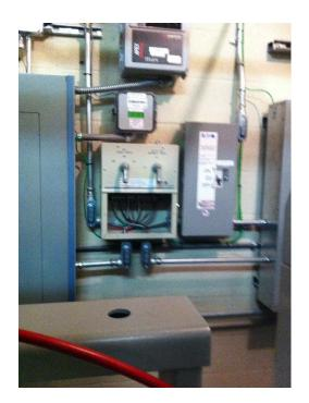
IMG\_1959 shows utility voltage as being a little low (well within specifications). This is probably due to the voltage loss in the overhead secondary line being about 300 feet long from the utility pole mounted transformer to the building.
