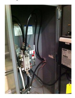
IMG\_1954 is a rough picture of the ATS system layout.
