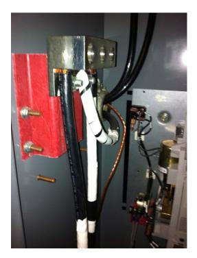
IMG\_1951 is a picture of the generator connections to the Switch. I did put a wrench to the closest ones and they were sufficiently tight.
