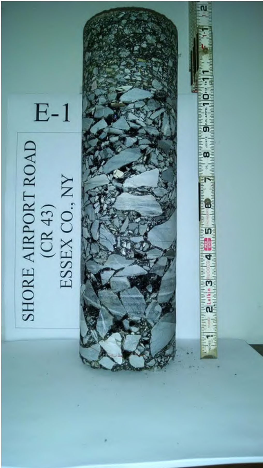
Pavement core at E-1 (in northbound travel lane)
