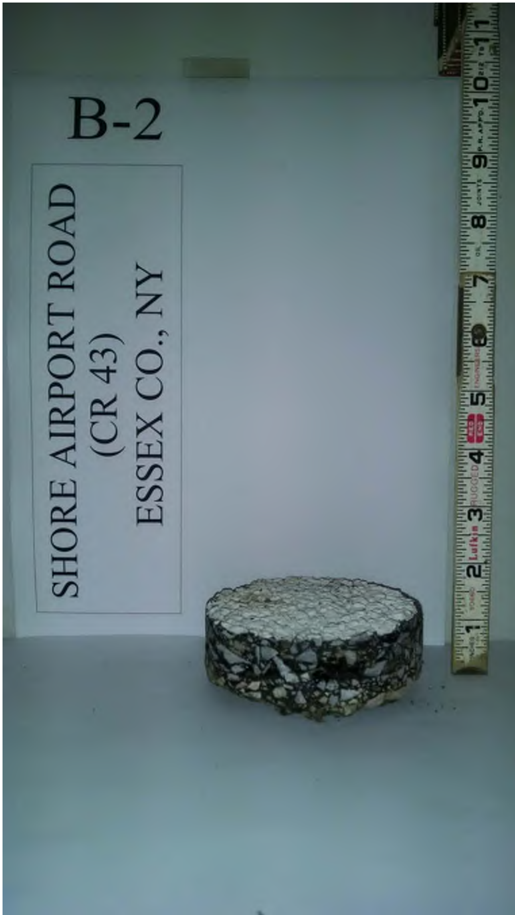
Pavement core at B-2 (in northbound shoulder)
