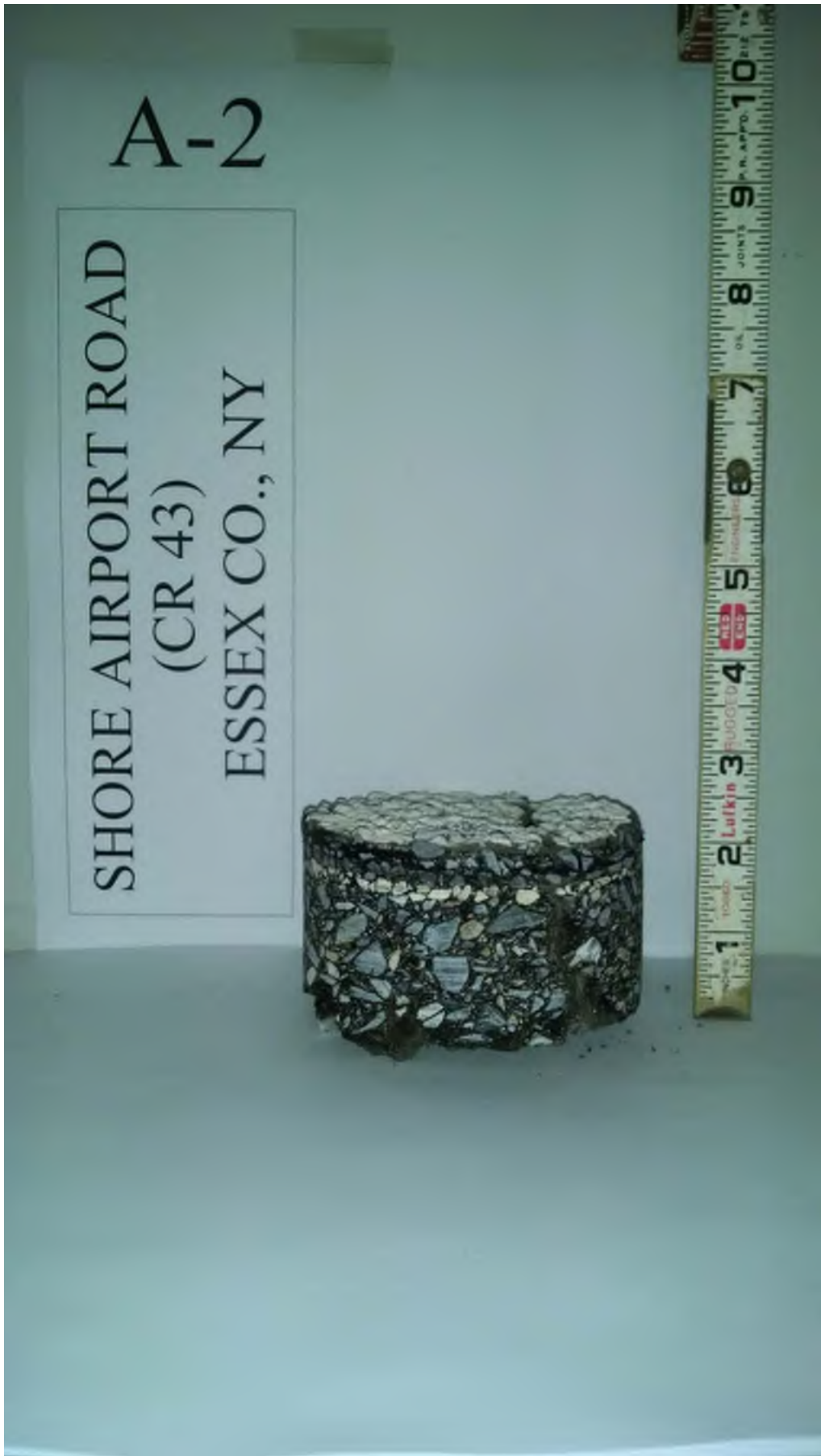
Pavement core at A-2 (in northbound shoulder)
