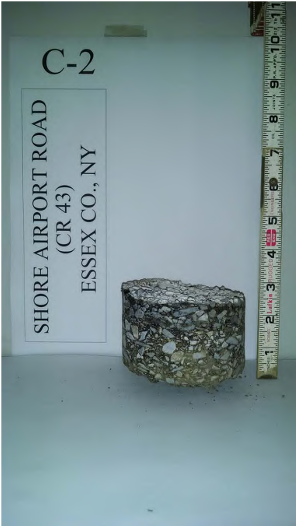
Pavement core at C-2 (in northbound shoulder)
