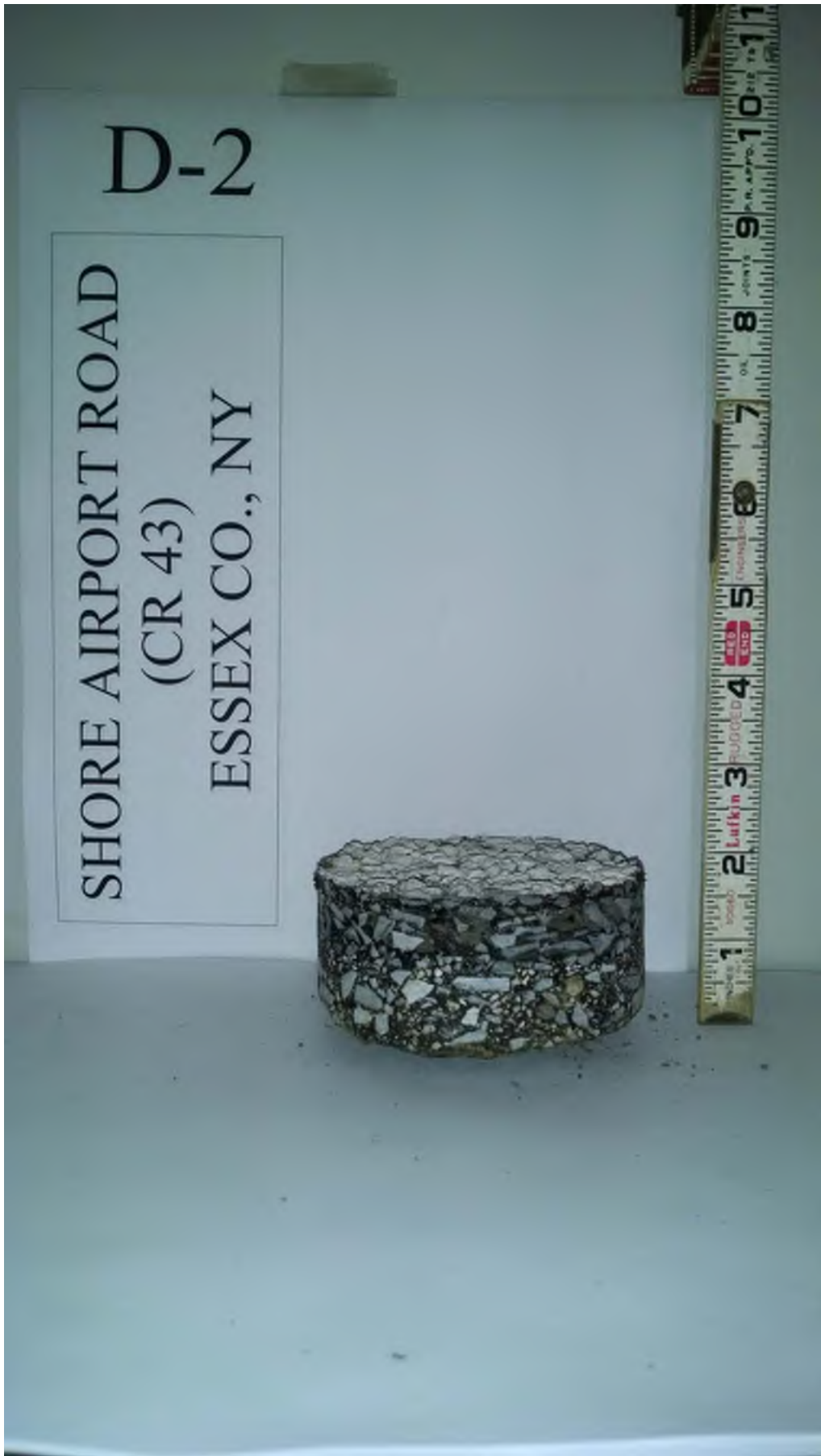
Pavement core at D-2 (in northbound shoulder)
