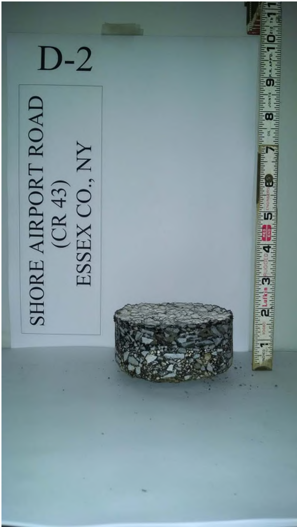
Pavement core at D-2 (in northbound shoulder)
