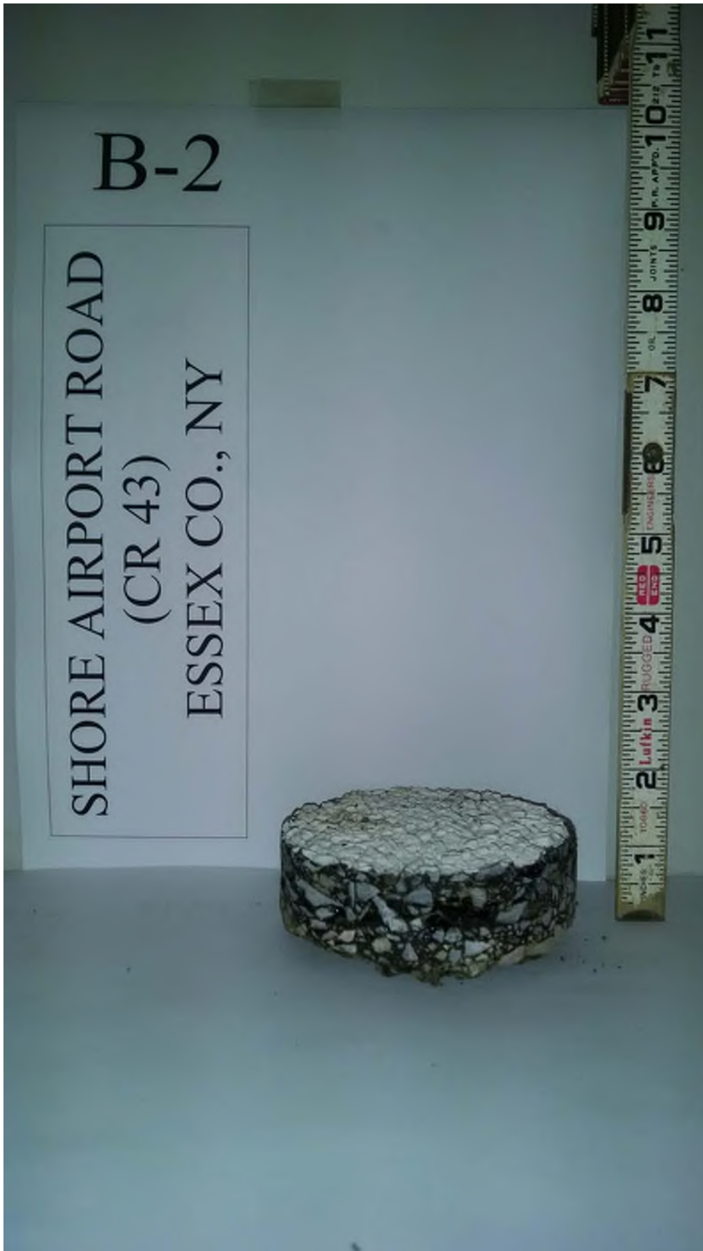
Pavement core at B-2 (in northbound shoulder)
