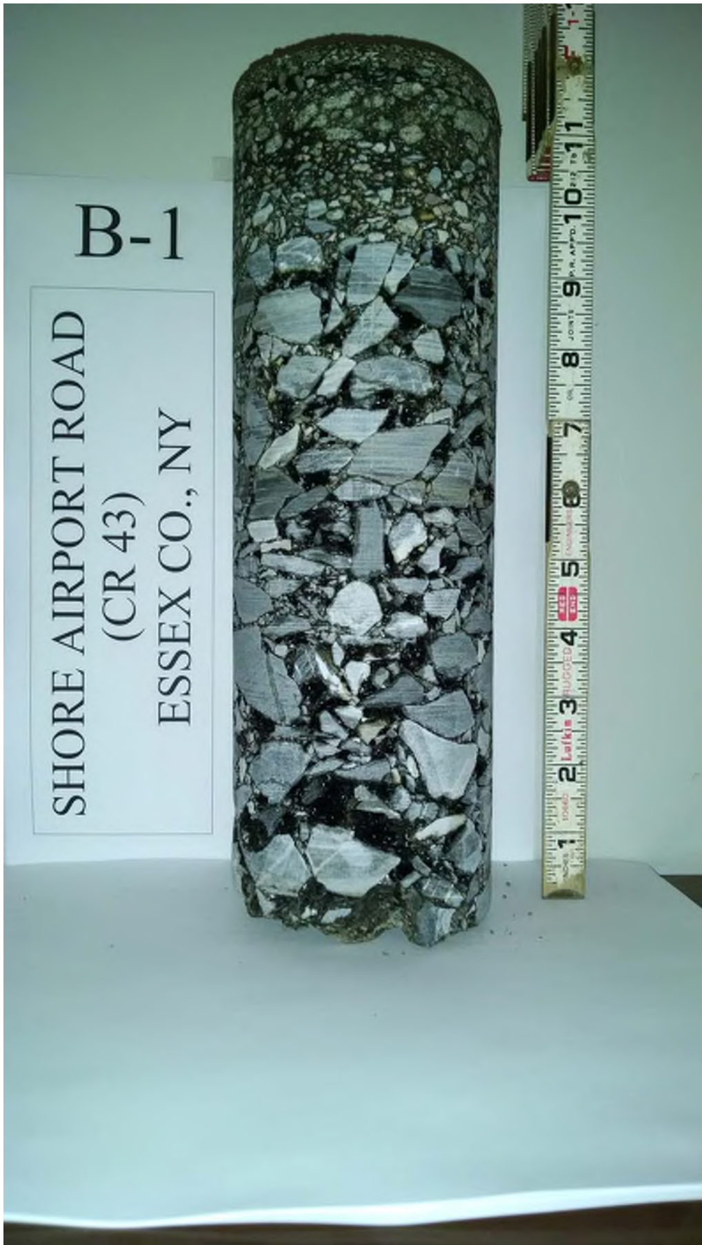
Pavement core at B-1 (in northbound travel lane)
