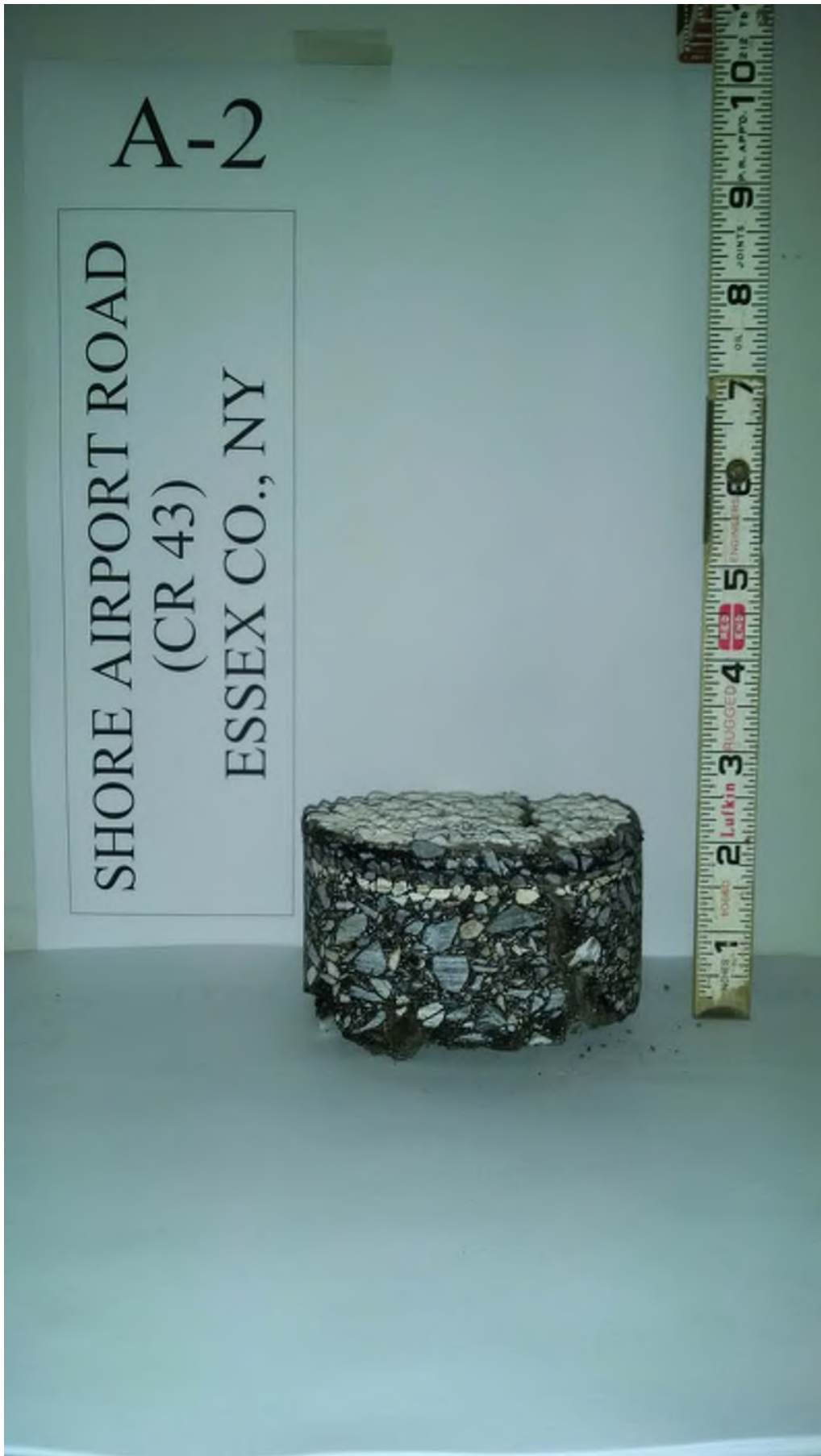
Pavement core at A-2 (in northbound shoulder)
