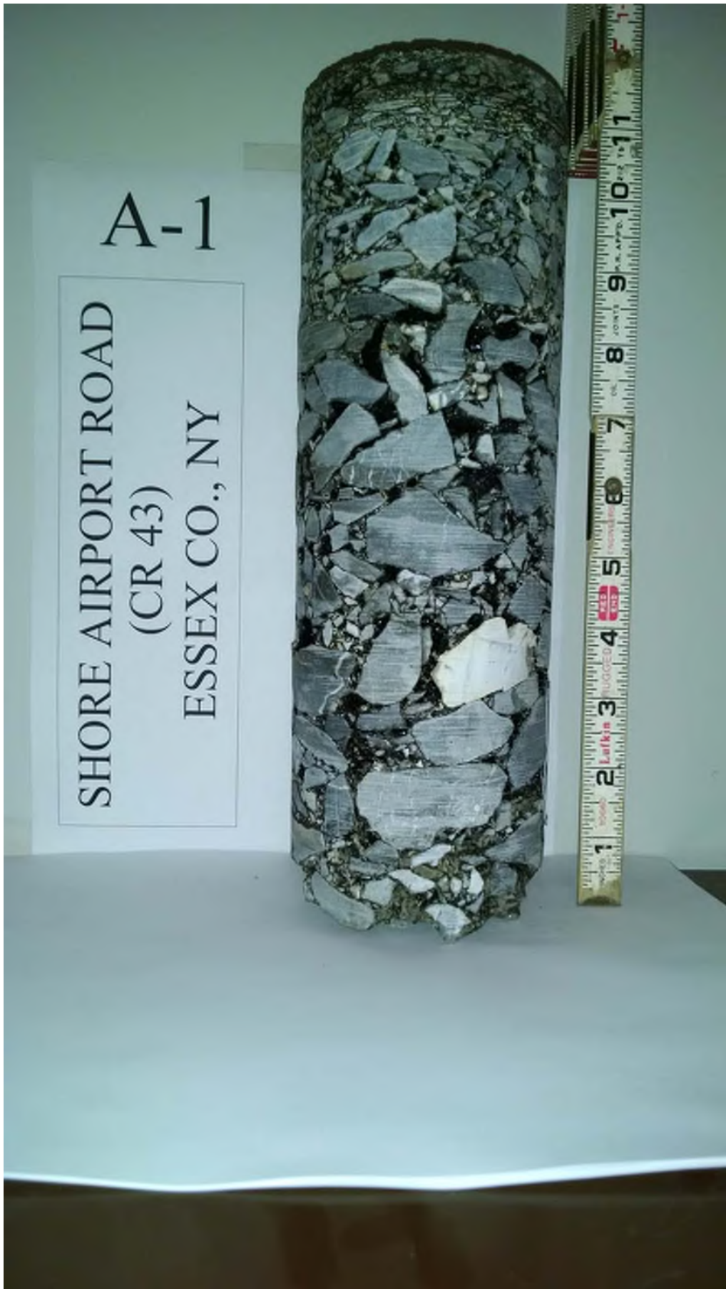
Pavement core at A-1 (in northbound travel lane)
