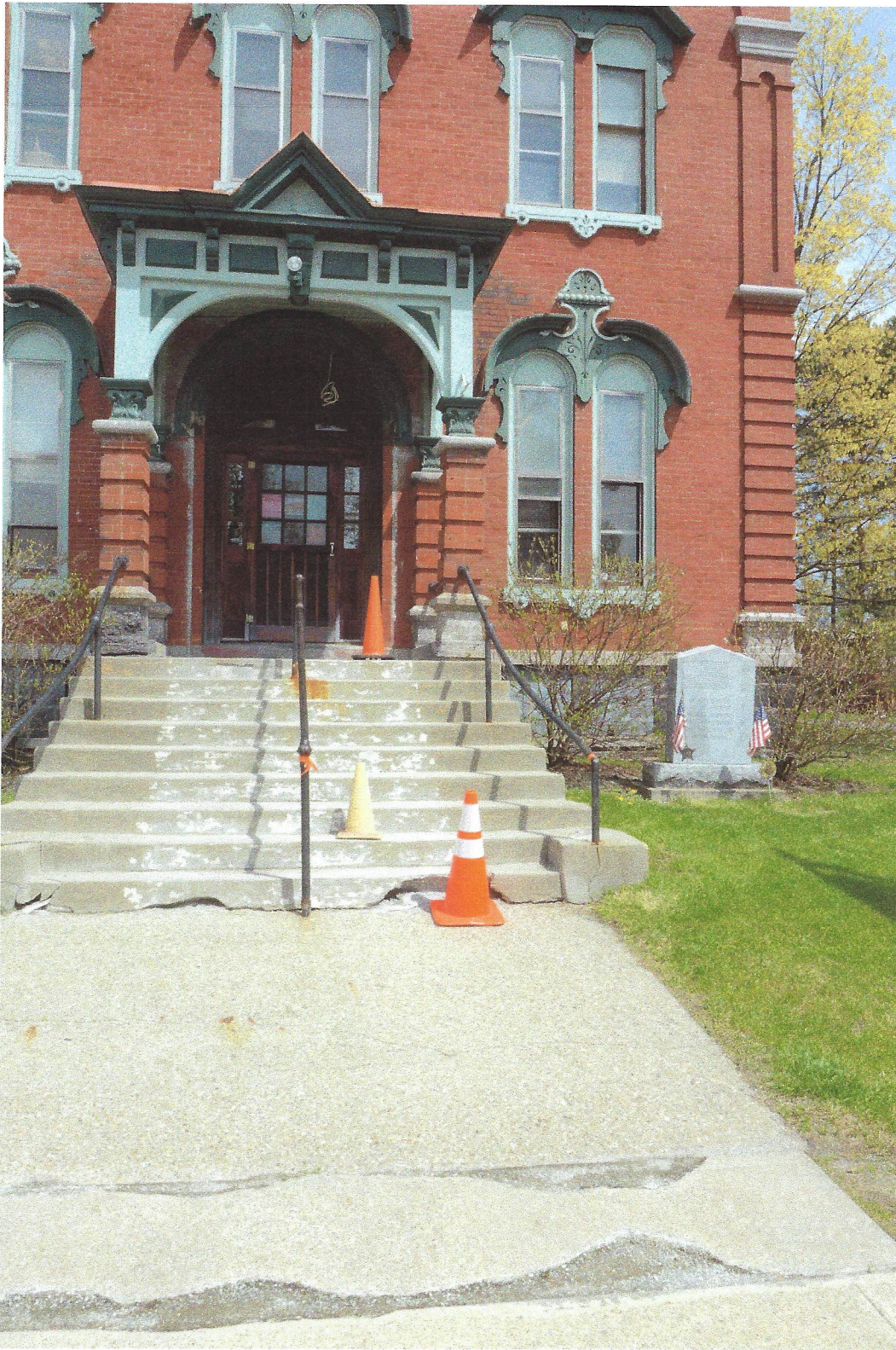
Main entrance stair to be refurbished
