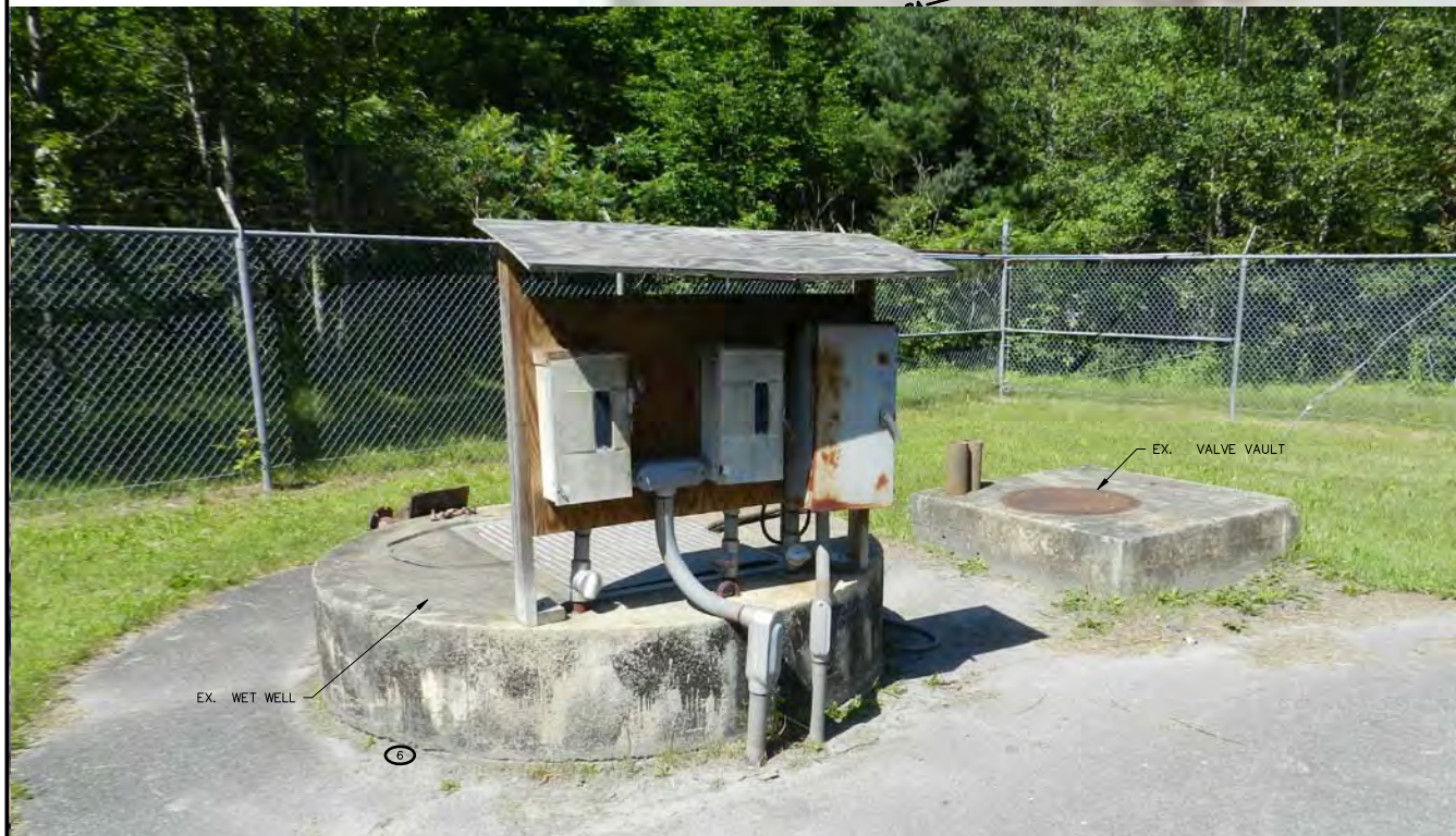
2 EX. WETWELL AND VALVE VAULT C-101 N.T.S.
