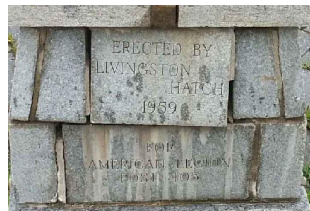
EXISTING DEDICATION PLAQUES
