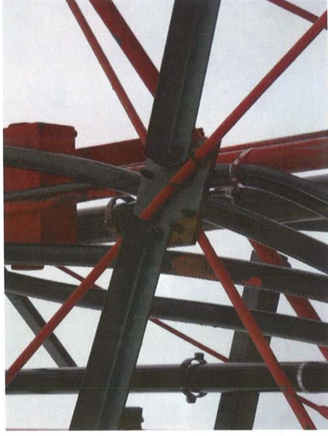
Exterior view of recent sub-brace connection to rod bracing.
