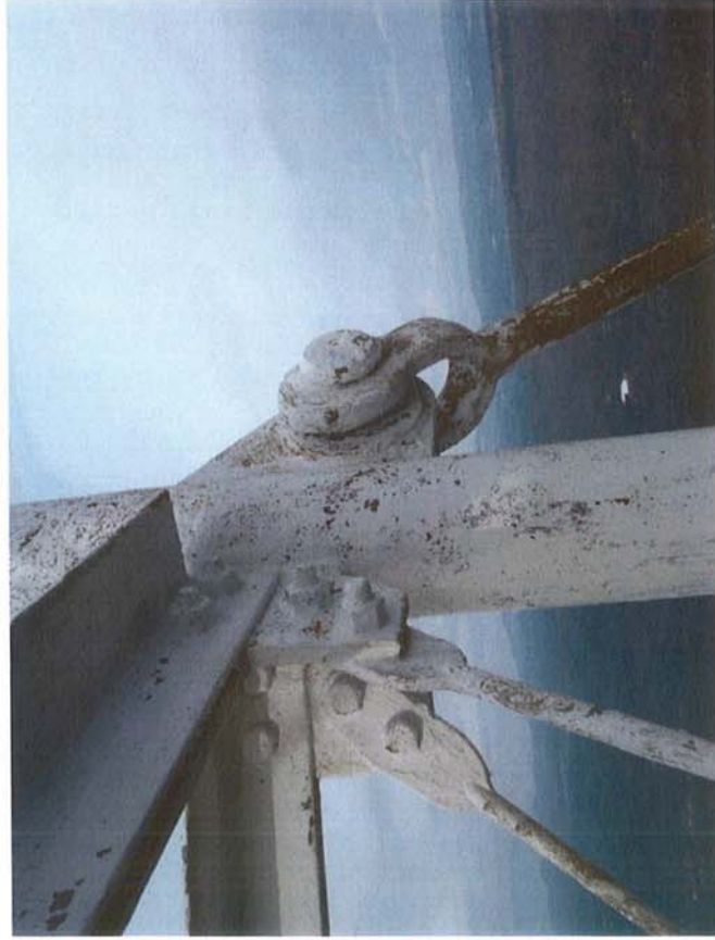
Guy connection co-located with brace point connection.
