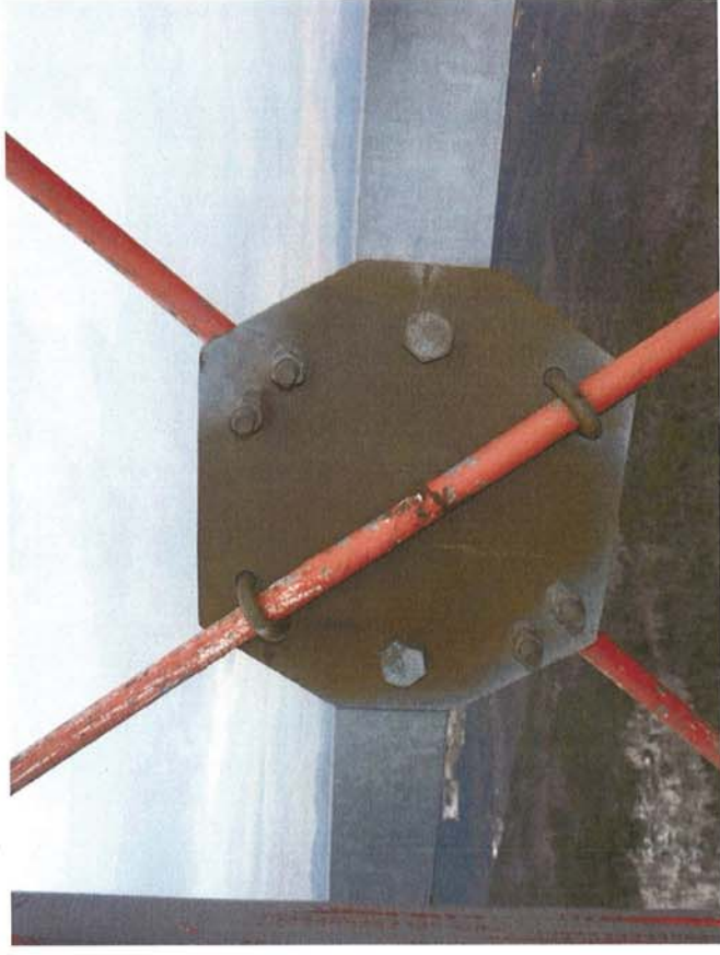
Interior view of recent sub-brace connection to rod bracing.
