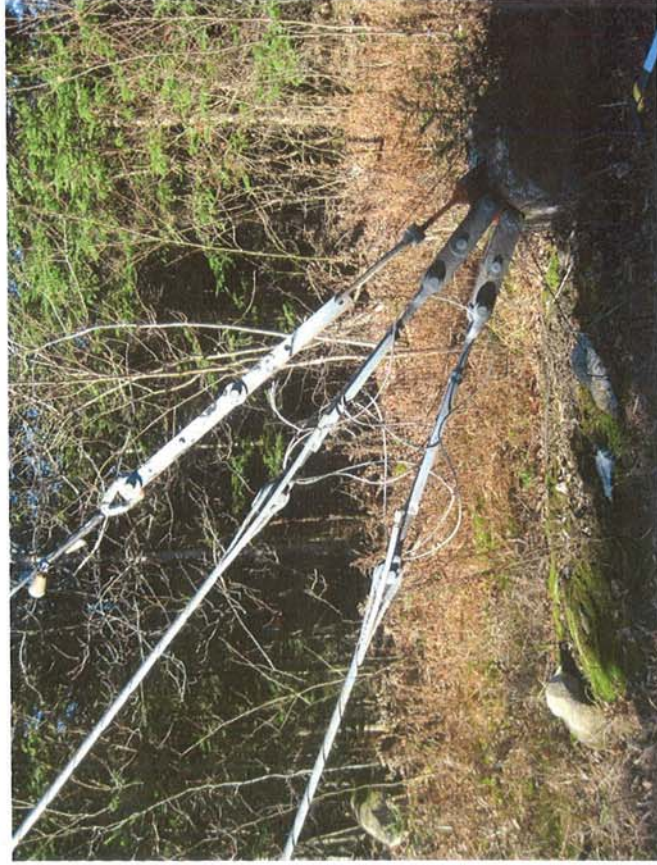
Typical lower level guy attachment point.
