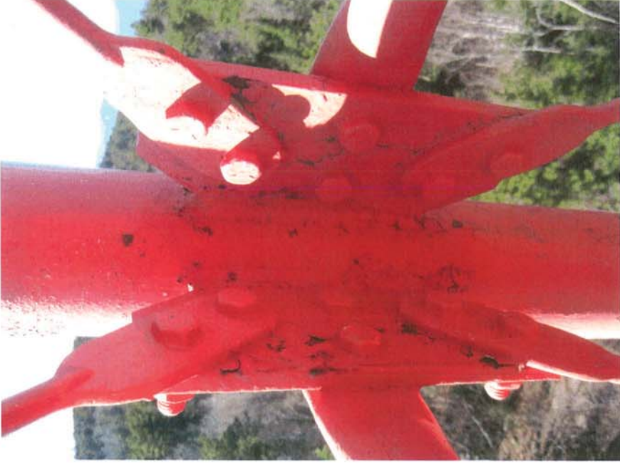
Typical horizontal and diagonal brace connection to leg.
