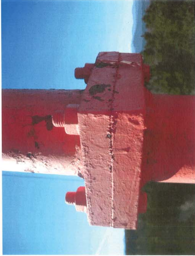
Typical leg section connection.
