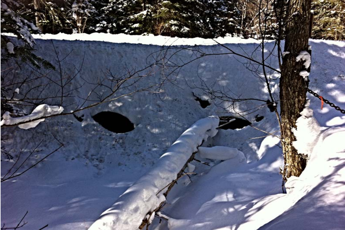
View of upstream bridge elevation
