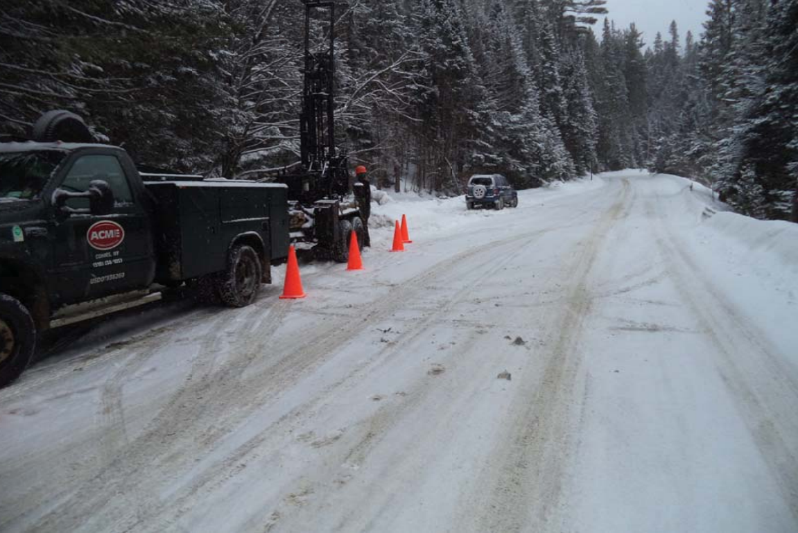
View south across culvert/bridge area
