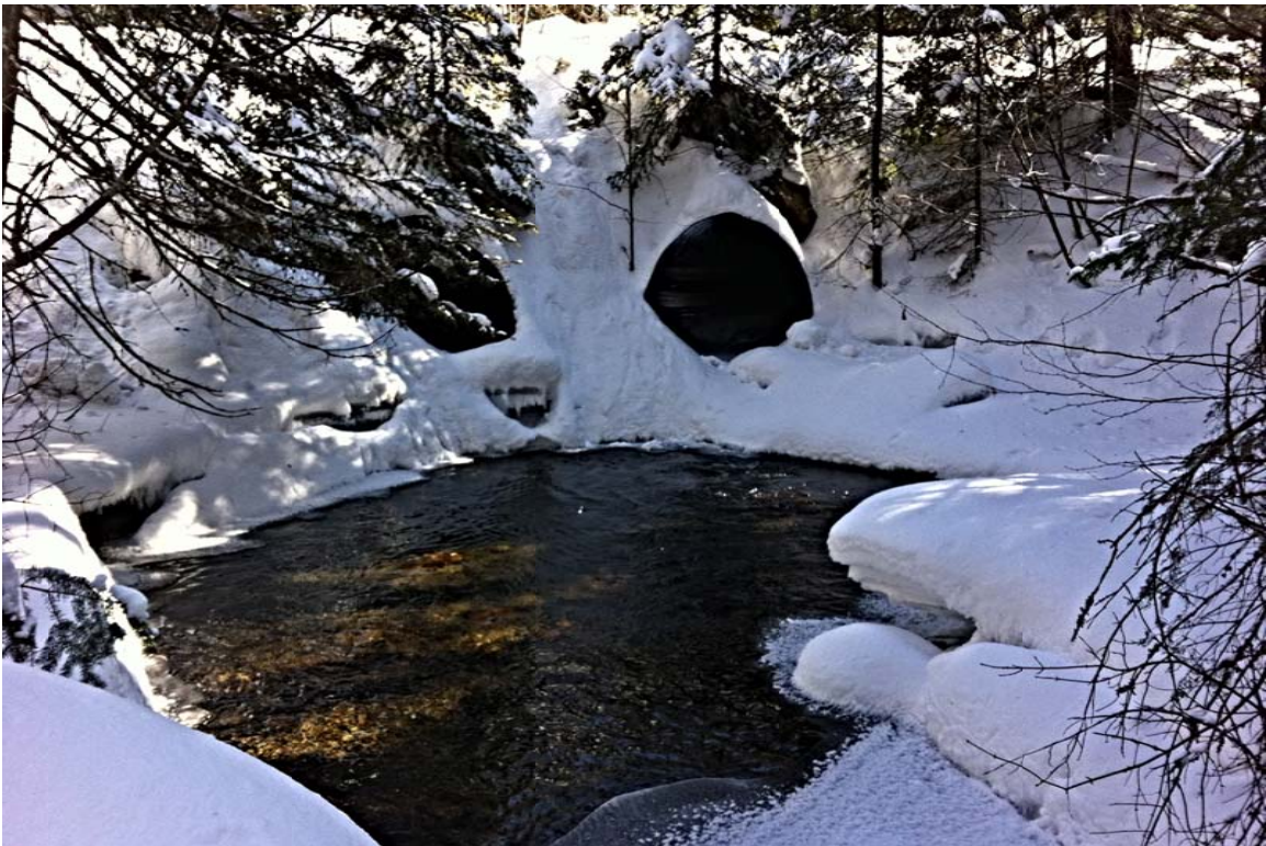
View of downstream bridge elevation
