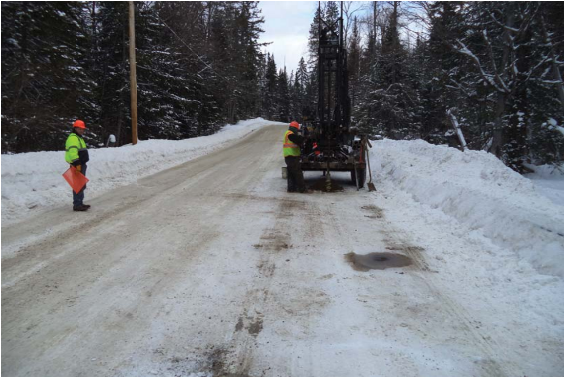
View northeast toward B-2 locations
